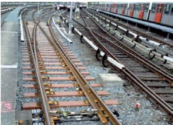
The modular turnout with synthetic sleepers was installed at HHA's Farmsen depot in less than one day.
