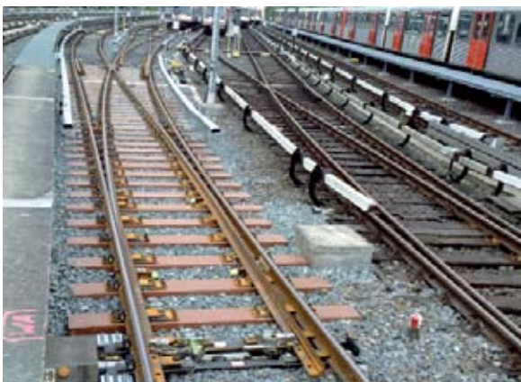
The modular turnout with synthetic sleepers was installed at HHA's Farmsen depot in less than one day.
