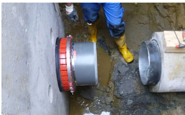
Fitting a sewer pipe to the BSM-Adapter®
