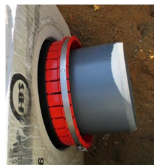
Inserting the BSM-Adapter® into the chamber socket
